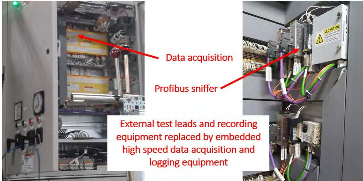
**Figure 5** Production Units Benefit from Embedded Data Acquisition and Logging Functions
