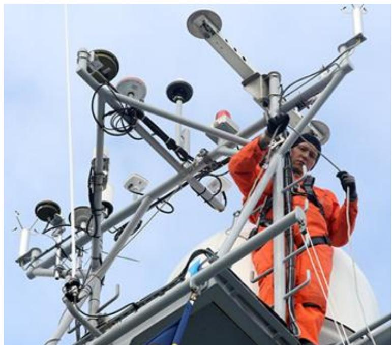
Figure 4: Example of complex antenna installation
