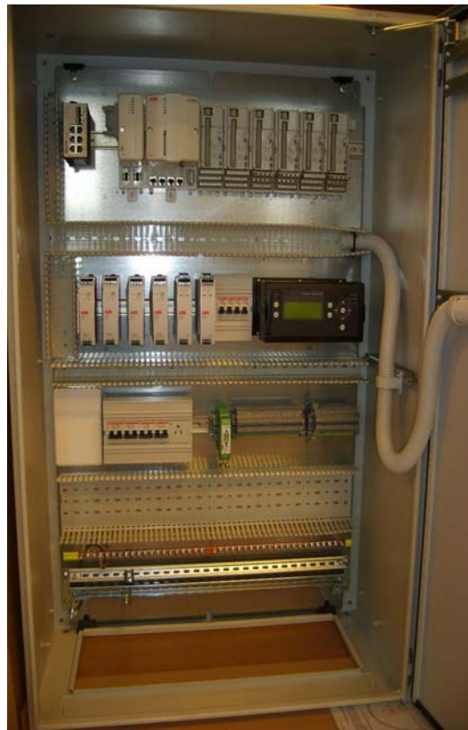
Figure 4: DGMS cabinet with standard dimension of 830 x 410 x 1140mm (LxWxH)
