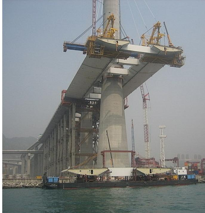
**Figure 2 – bridge segment on barge**
