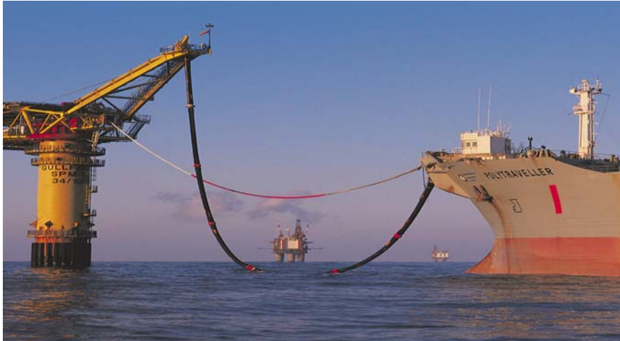
SPM loading at Gullfaks field.
